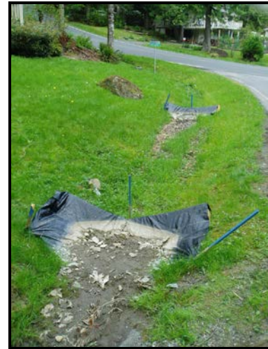
Triangular Silt Dike
