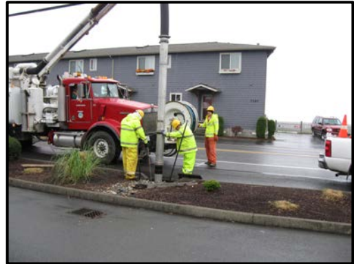
Catch basin cleaning in Birch Bay
