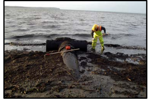
Stormwater outfall cleaning in Birch Bay
